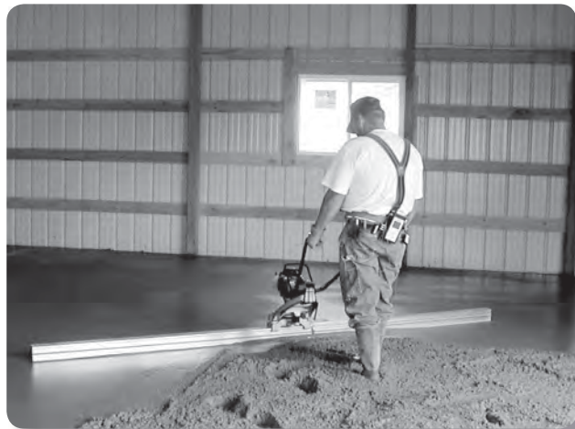
Solution: Motorized screeding
