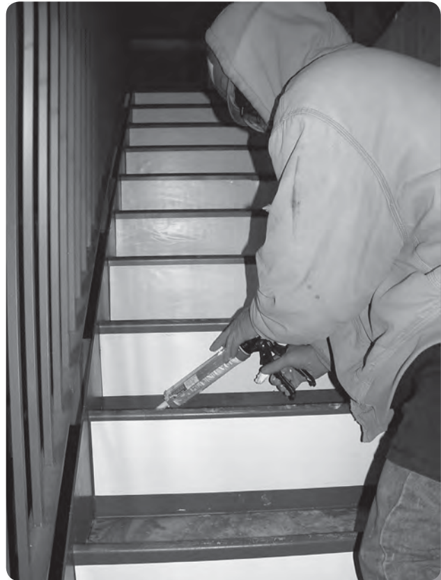
Problem: Manually squeezing caulking gun
