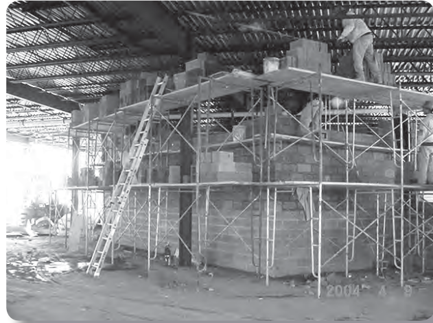
Problem: Conventional unguarded frame scaffolding
