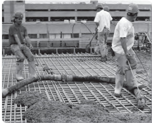
Problem: Pulling concrete hose without skid plate
