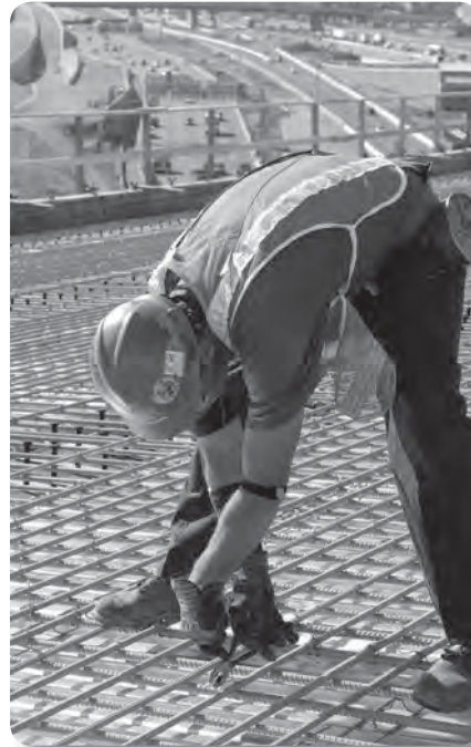
Problem: Tying rebar by hand
