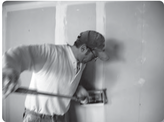
Problem: Hand drywall finishing with mudbox
