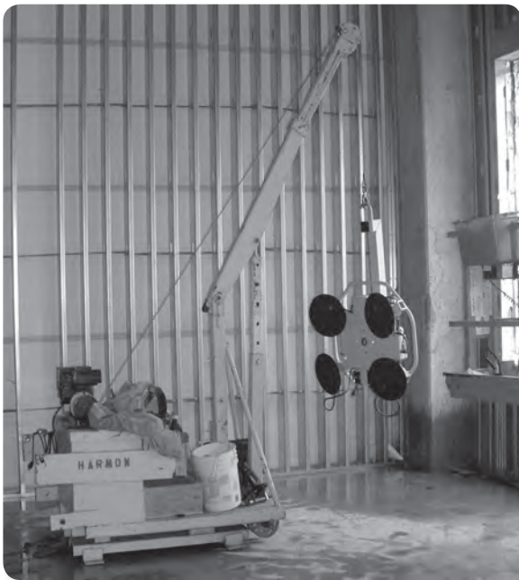
Power vacuum lifter avoids manual lifting
