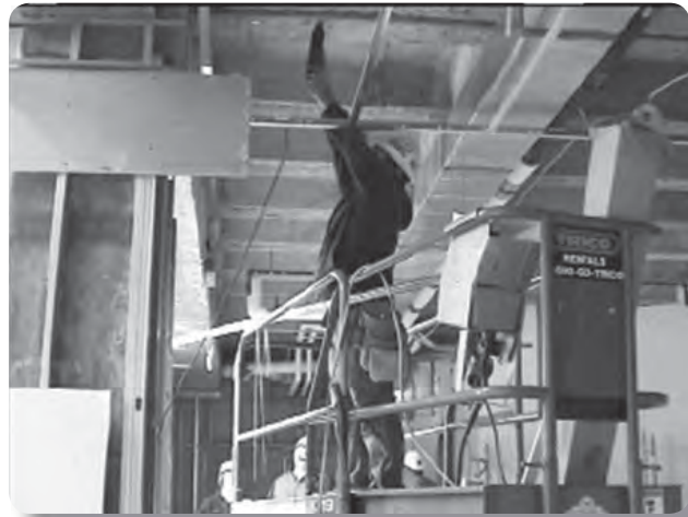
Problem: Drilling overhead
