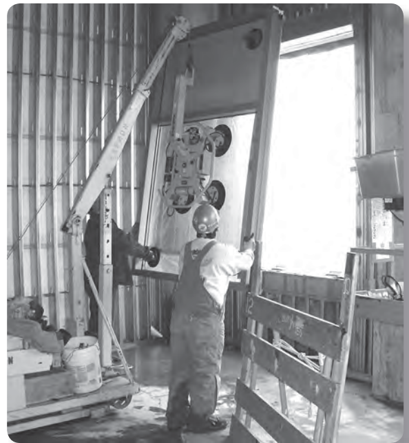
Power vacuum lifter avoids manual lifting
