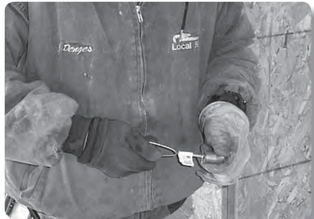
Problem: Brushing copper tube by hand
