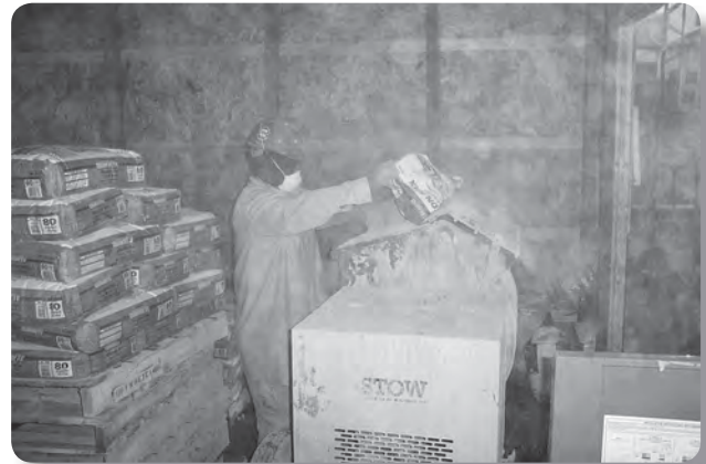
Problem: Traditional method of loading mixer
