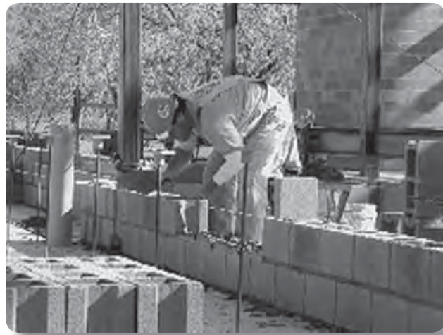
Problem: Laying standard concrete block
